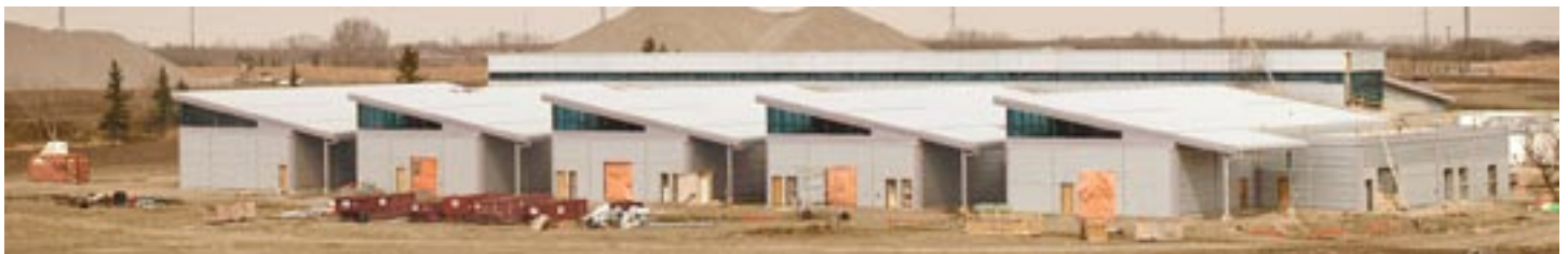
New Clinical Skills Building (under construction)
